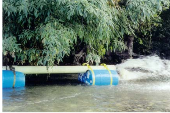
Picture 3. Discharge pipe with barrels attached
