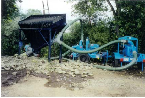
Picture 2. Two 6-inch water pumps and hopper
